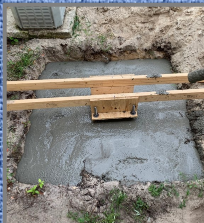
Cement was poured in the holes.
